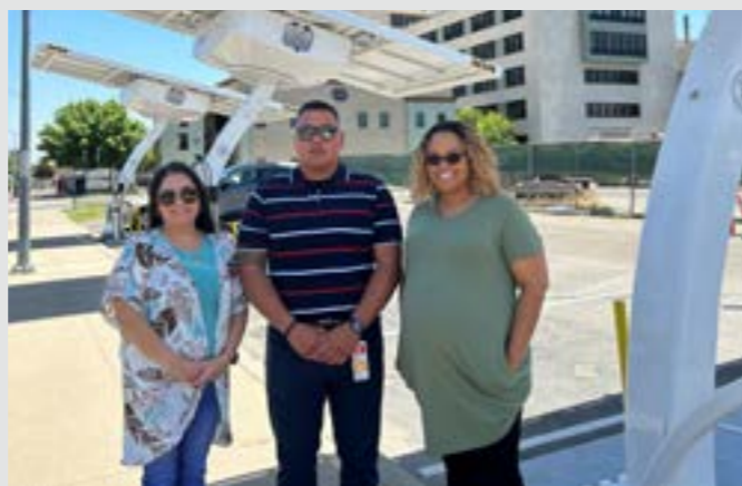
Three solar-powered electric vehicle (EV) charging stations were delivered to the campus on June 28. VACCHCS is also working to implement a composting program by the beginning of 2024 to comply with new state regulations.
